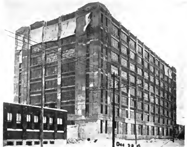
BUILDING FOR ROBERT SIMPSON CO., LTD., REGINA, SASKATCHEWAN. VIEW TAKEN DURING CONSTRUCTION
